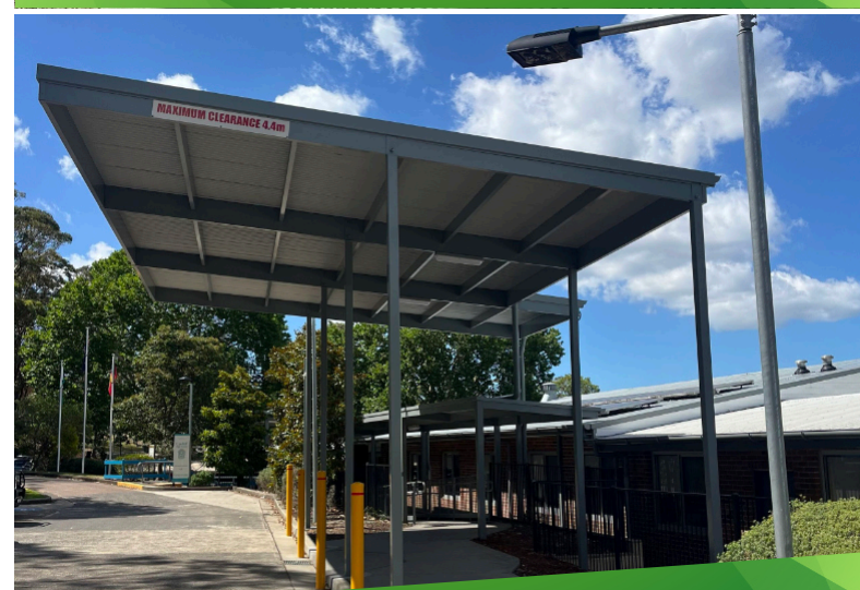
BUS BAY SHELTERS
